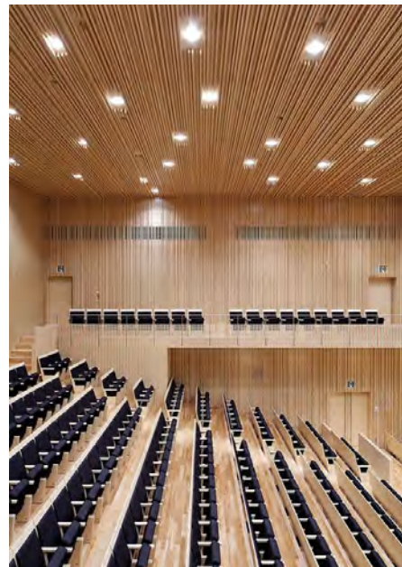
Timber strip ceiling
